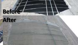
Large Repair on Concrete Stack
